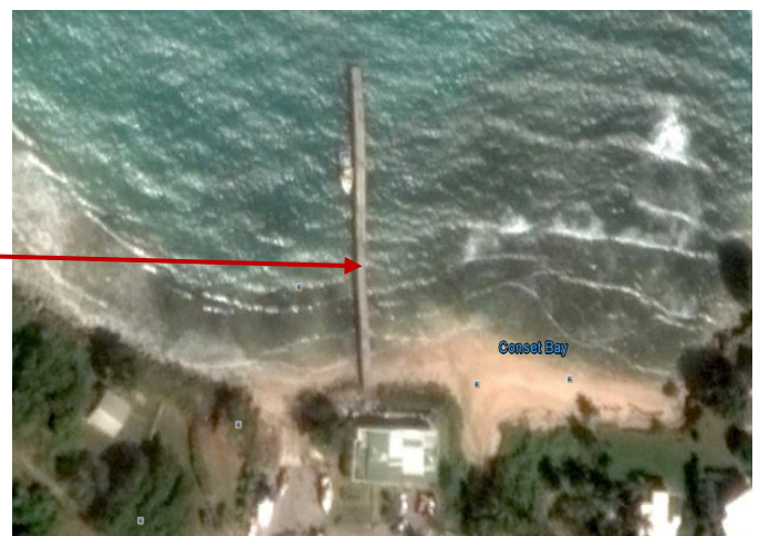
FIGURE 3: RADAR SENSOR LOCATION – CONSETT BAY, ST. JOHN
