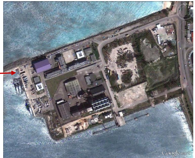
FIGURE 2: RADAR SENSOR LOCATION – BARBADOS COAST GUARD
